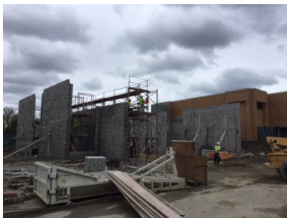
Sprague – Masonry Walls
