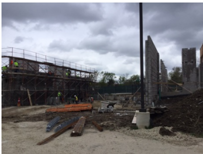
Sprague –Masonry Walls
