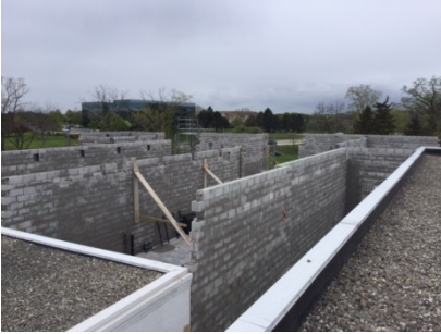
Half Day – Level 2 Masonry Walls
