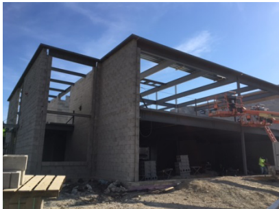
Sprague – Steel in place, view from SW
