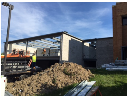
Sprague – Steel in place, view from SE
