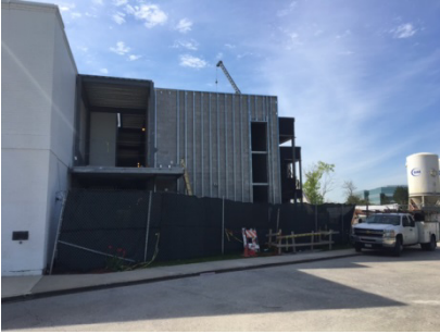
Half Day – North Side Exterior Wall
