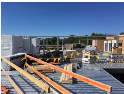
Sprague – Rooftop Equipment
