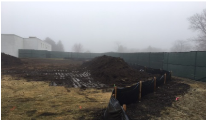
Half Day Site Clearing
