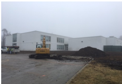
Half Day Site Clearing
