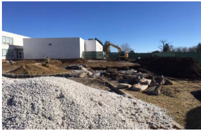
Half Day – Excavation
