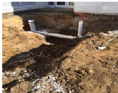
Half Day – Underground Utilities
