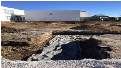
Half Day – Excavation
