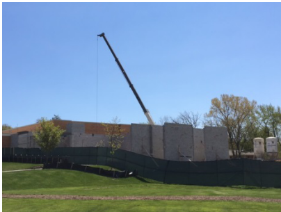
Sprague – Structural Steel Installation
