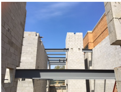
Sprague – Steel in place
