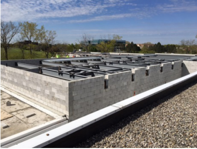
Half Day – Level 2 Structural Steel
