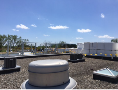
Half Day – Roofing in Progress
