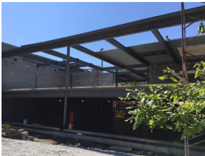
Sprague – Roof Steel Decking Installation
