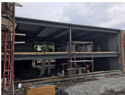
Sprague – Structural Steel
