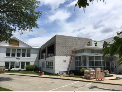
Half Day – Exterior, 2 nd Floor Addition
