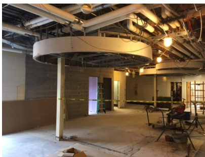
Sprague – Interior, Renovated Space
