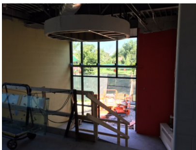
Sprague – North stair and entrance
