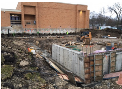
Sprague – Foundations at Northwest
