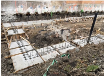
Sprague – Footings at Northeast
