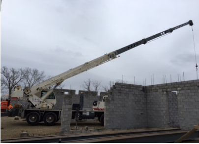
Half Day – Steel Erection
