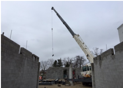
Half Day – Steel Erection
